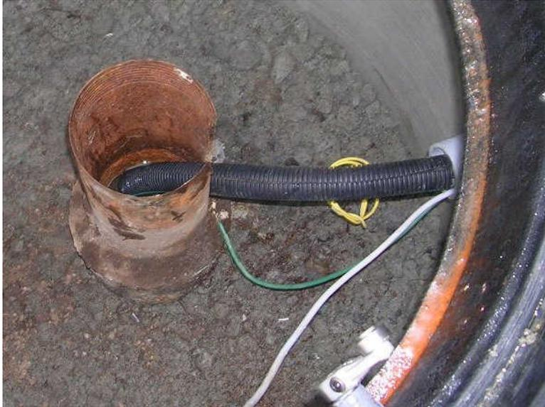
An earth strap can be used to ensure a good connection.
