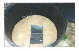
If you are installing in a cased pit (as in this picture), install the digitizer and power supply inside if possible, and seal the installation with a weatherproof cover.
