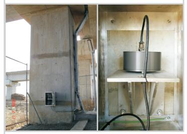
This new project, comprising 80 Güralp strong-motion accelerometers, gathers real-time data from structures along a newly-built high-speed railway line, and transmits it to operators using a combination of Scream! and DSS protocols.
