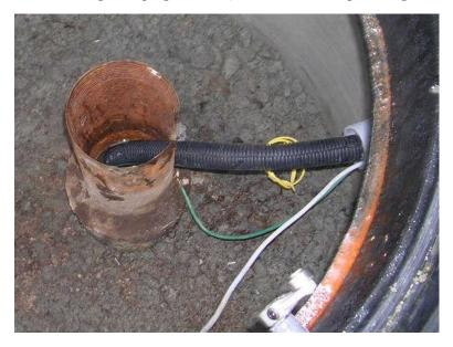
An earth strap can be used to ensure a good connection.
