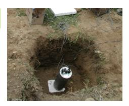
Connect the sensor cables, then level and unlock the components as described in steps 3 and 4 overleaf.
