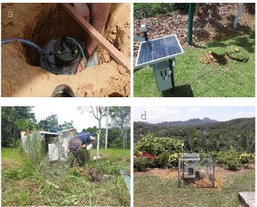
*Figure 5: Clockwise from top left: (a) installation of seismometer (b) solar powered transmitter (c) housing installation featuring local feline (d) completed station.*
