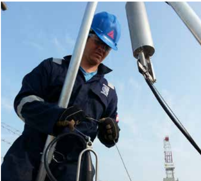
GÜRALP FIELD SERVICE ENGINEER INSTALLING A BOREHOLE STATION
