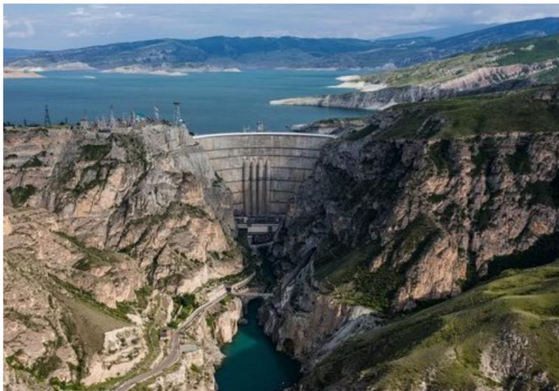
*Fig. 1 Chirkeisk Dam, Dagestan Republic, Russia. Although strong-motion sensors are already deployed on the dam, this project required an array of broadband seismometers to detect and characterise regional earthquakes.*
