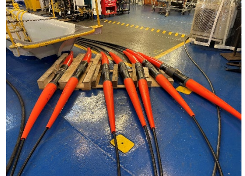
Image 5. The seven universal joints required to splice the repeaters into the cable
