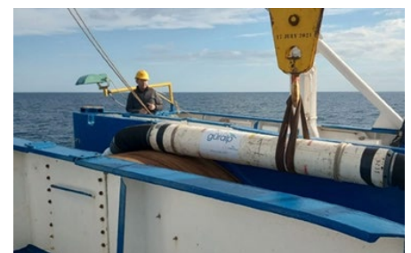
Image 7. Repeater being deployed
