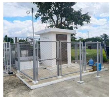
Figure 16 (left): A 3T deployment in a dedicated vault enclosure onto a concrete plinth installed onto bedrock.
