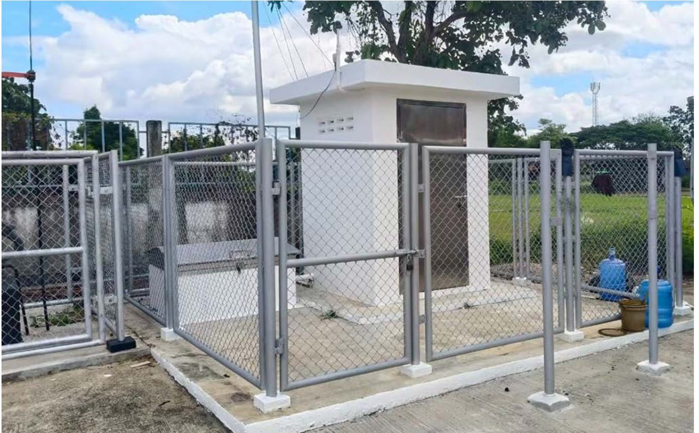
Figure 1: The exterior of one of the permanent monitoring stations
